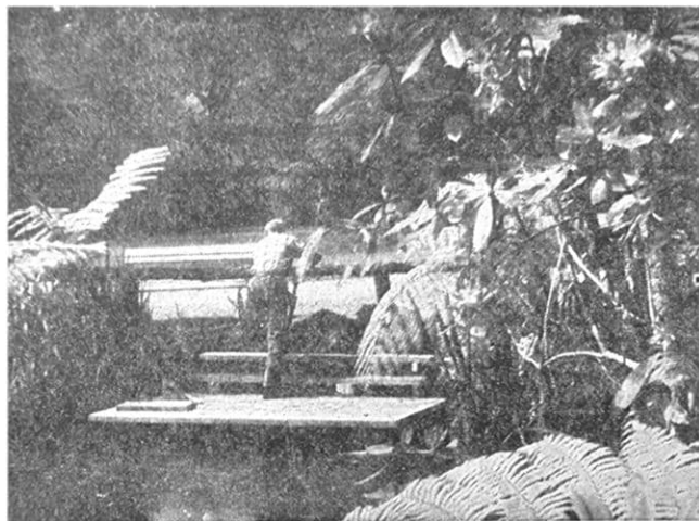
A MEMBER of the Pukekura Park staff, Mr. E. Powell, installs steps leading down to one of two wooden landings, which have been erected at the northern and southern ends of the fountain lake for a double purpose.
