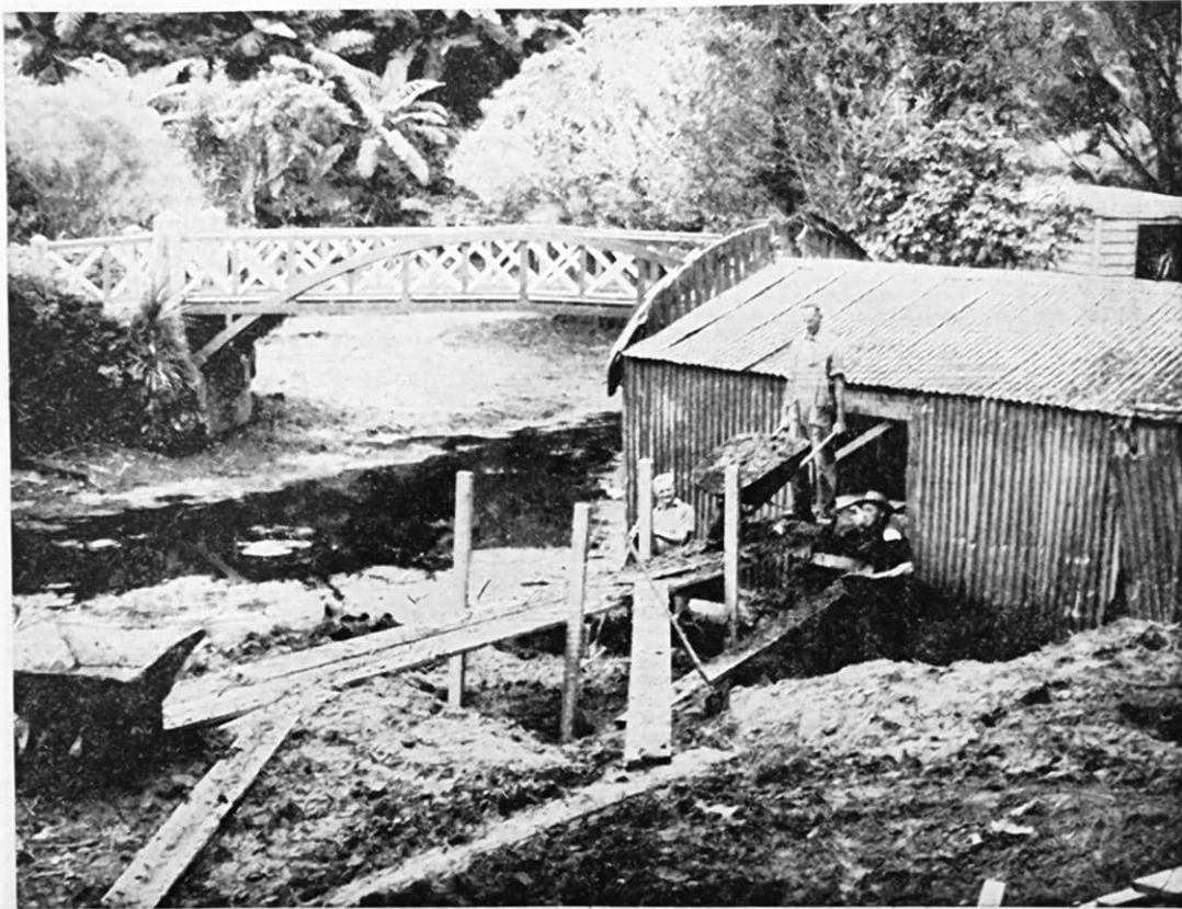
THE LEVEL of the main lake in Pukekura Park, New Plymouth, has been lowered about 4 feet 6 inches to allow work to begin on the site of the new boathouse. Members of the park staff are here seen removing soil from the area of the old boatshed. Some 220 cubic yards will have to be excavated before erection of the new building can begin. The upper, or boatshed, bridge is in the background.
